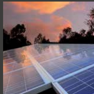
Attika-Blende und Photovoltaik
